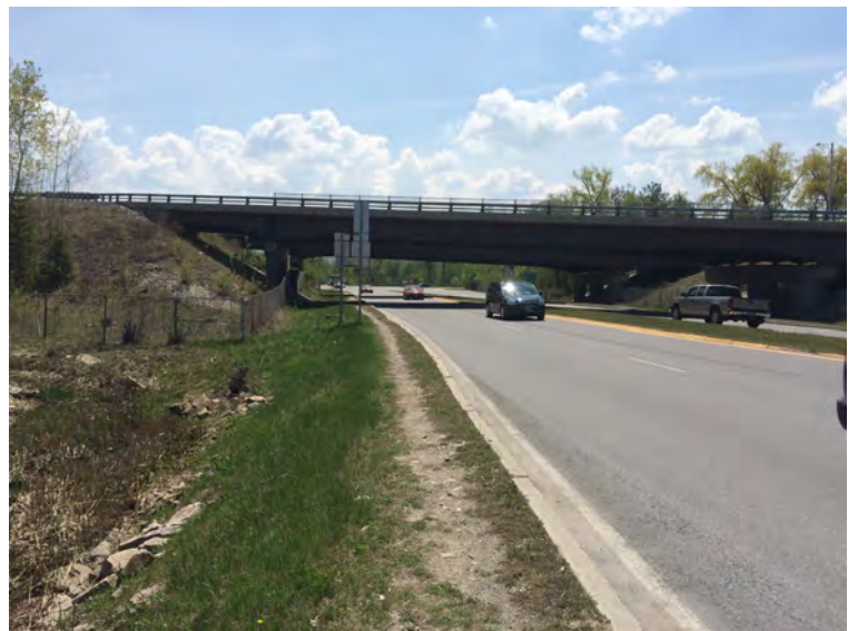
VT-279 overpass over VT67A and path of desire footpath.
