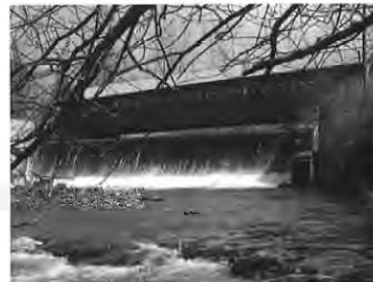
A local energy entrepreneur re-established the hydroelectric generating capacity at the “Paper Mill” site along the Walloomsac River in Bennington. The facility is rated at 360KW generating capacity and produces electricity with greater consistency and reliability than solar or wind facilities.
